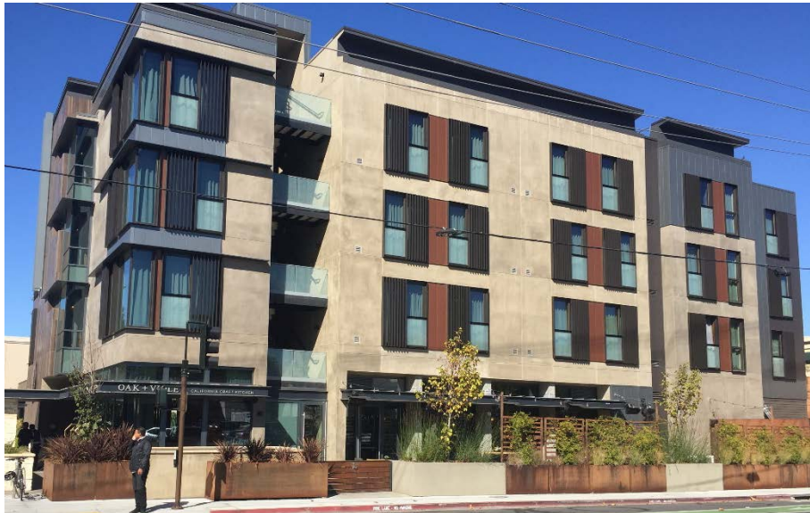
FIGURE S.0.1-3 Hybrid Construction; View of Finished Building (P1415) In this hotel, the large ground level restaurant serving a popular area, and the parking levels below grade called for wide open spans. The post-tensioned podium slab over the ground level supports the light framed hotel rooms with short spans and multitude of non-aligned walls with the ground level supports.
